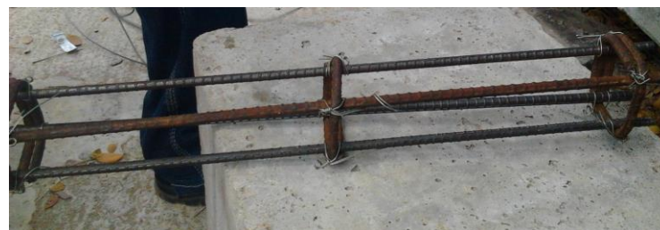
Figure 2.2: Reinforcement bar before winding
