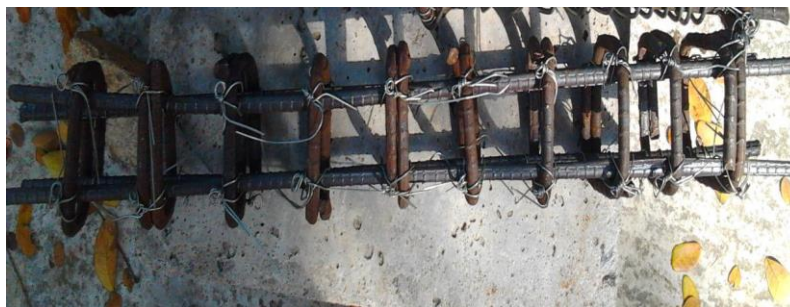
Figure 2.5: Beam with normal 6mm stirrups
