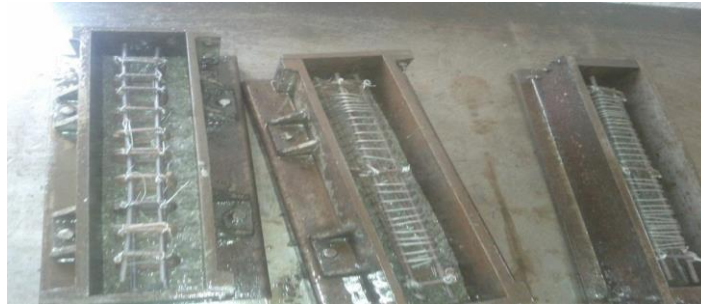
Figure 3.1: casting of beam with normal stirrups and 3mm wire spiral stirrups
